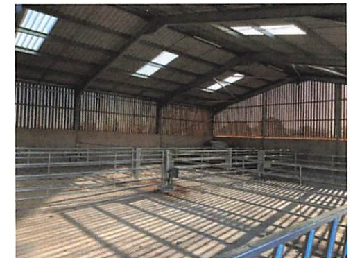
New Farm Building
